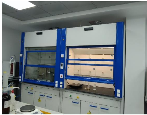
2023 – NEW INNOVATIVE CO. (Yanbu) Blower Fan Supply & Installation
